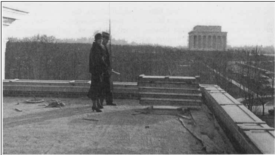
On top of the Pharmacy Headquarters Building. This view shows the proximity of the building to Lincoln Memorial. Daughter of Treasurer Charles W. Holton and Secretary E. F. Kelly are taking in the situation.
